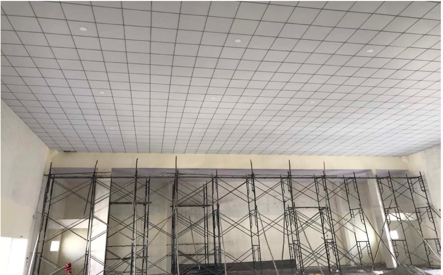
PVC false ceiling with LED lights and side walls being plastered
